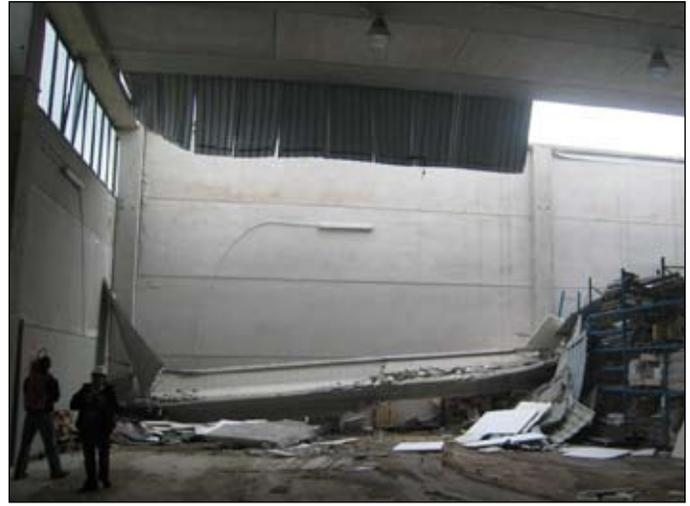
**Figure 18.** Partial collapse of the roof.
