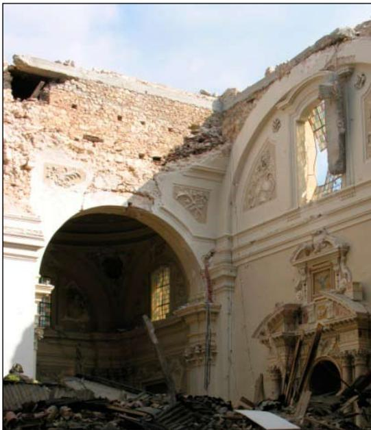
**Figure 10.** Roof and cupola collapse in the Santa Maria di Collemaggio Abbey in L'Aquila. The reinforced concrete ring beam did not prevent the collapse of the cupola.
