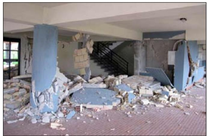
**Figure 14.** Core shear wall with extensive structural damage and failure in a modern RC building in Pettino.
