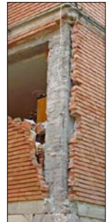
**Figure 11a/b.** Typical damage to infill walls.
