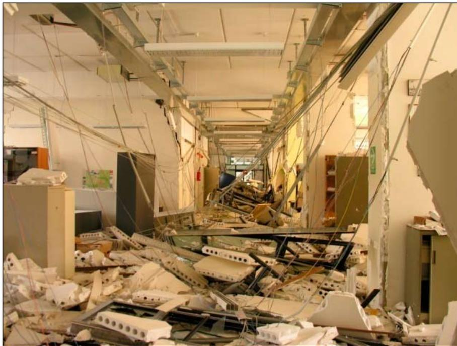
**Figure 15.** The interior of the City Planning Offices in L'Aquila. Note that the building exterior has very minor detectable damage.
