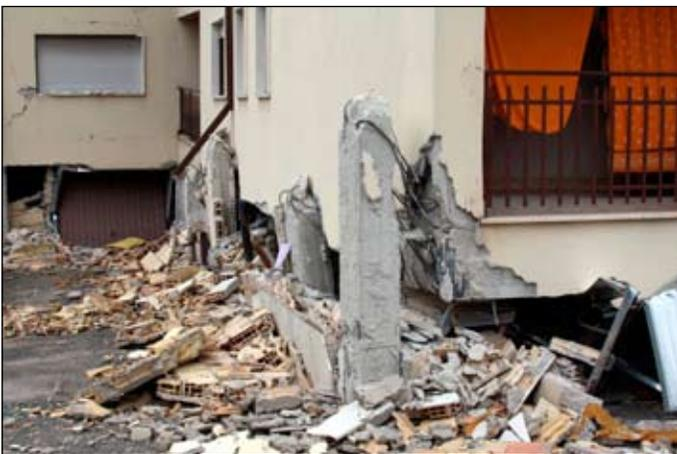
**Figure 13.** Soft-story collapse in Pettino. Two of four almost identical structures collapsed.
