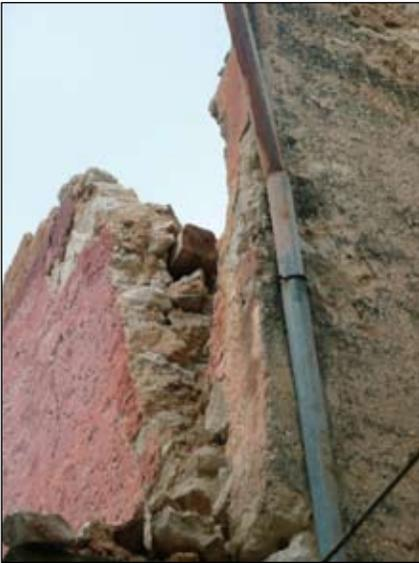
**Figure 7.** Detail of 18th century wall-strengthening system, where no ties connect the beam to the wall.
