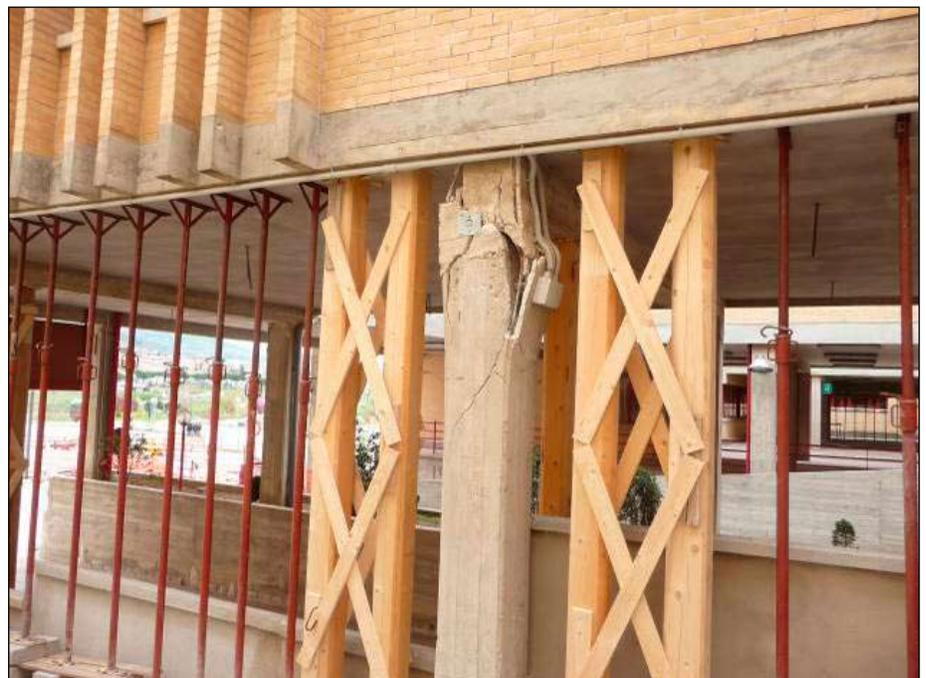
**Figure 16.** Column damage at hospital entry structure; no tie reinforcement is evident.
