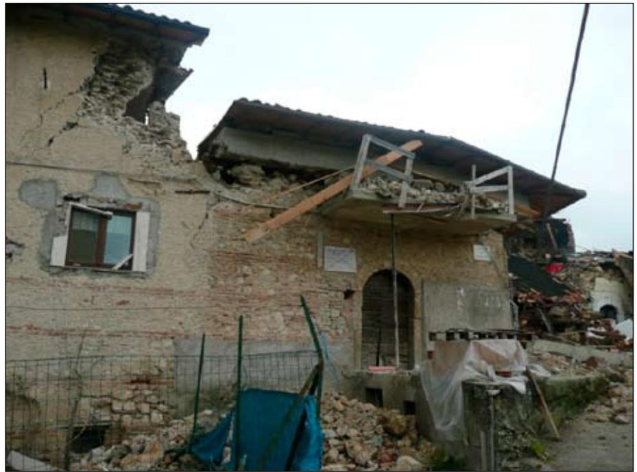
**Figure 8.** Collapse of a masonry building in Temperra with concrete ring beam retrofit.
