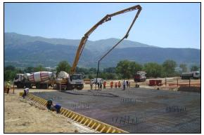
Figure 17 The base pad for the temporary housing units was being filled with concrete. There were three pads on this site.
