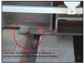
Figure 5 Steel angles were welded to prevent the transformers in substations from sliding after the earthquake.
