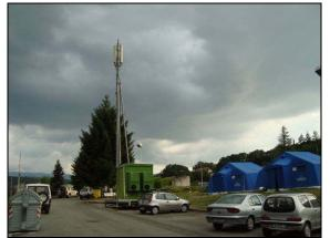
Figure 7 Many temporary cell sites like this shown were set up to compliment the landline communication service.
