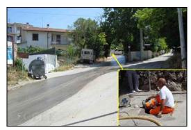
Figure 11 A water valve in a manhole was being repaired in Paganica.
