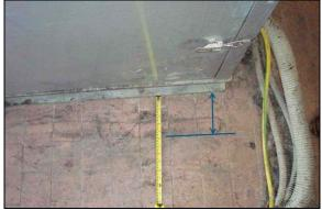
Figure 14 The pump in the control room of the new wastewater treatment plant was not anchored and shifted during the earthquake. It shifted about 15 cm.
