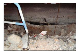
Figure 8 Underground telecommunication landlines were damaged and being repaired.
