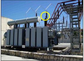
Figure 1. The rigid bus connection at the top of the transformer was damaged during the earthquake.
