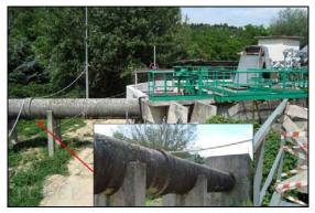
Figure 13 The waste intake pipe at the old treatment plant was dislocated at the joint, leaking dirt water.
