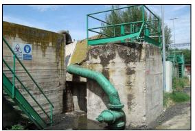
Figure 12 This aeration tank in the old wastewater treatment plant was damaged. Note the wall of the tank collapsed. The dirt water spilled all over.
