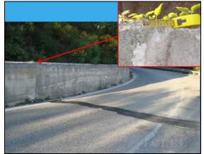
Figure 9 Some part of the State highway SS80 was damaged, this shows the displacement of the retaining wall and surface crack on the road surface. The offset was about 9 cm.
