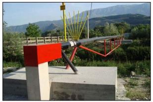
Figure 15 This new gas pipeline replaced the old damaged one in Onna. Note that the pipe is fixed on the concrete block.
