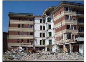
Figure 16 The student dormitory was severely damaged with one part collapsed.
