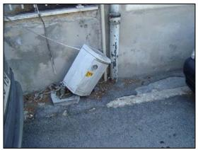
Figure 2 A lot of this type of low voltage distribution connection boxes was damaged resulting in power interruption.
