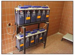
Figure 6 Unanchored battery racks and the batteries on the racks were not secured were common in substation control rooms.
