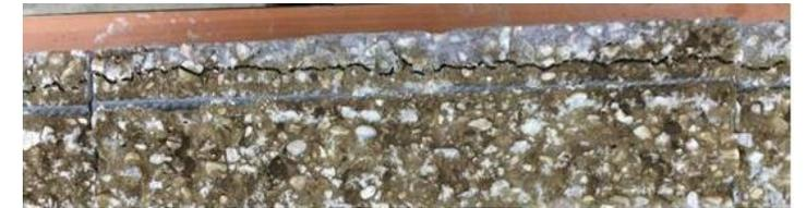
Chloride ingress due to diffusion through the concrete cover in a beam without bending cracks
