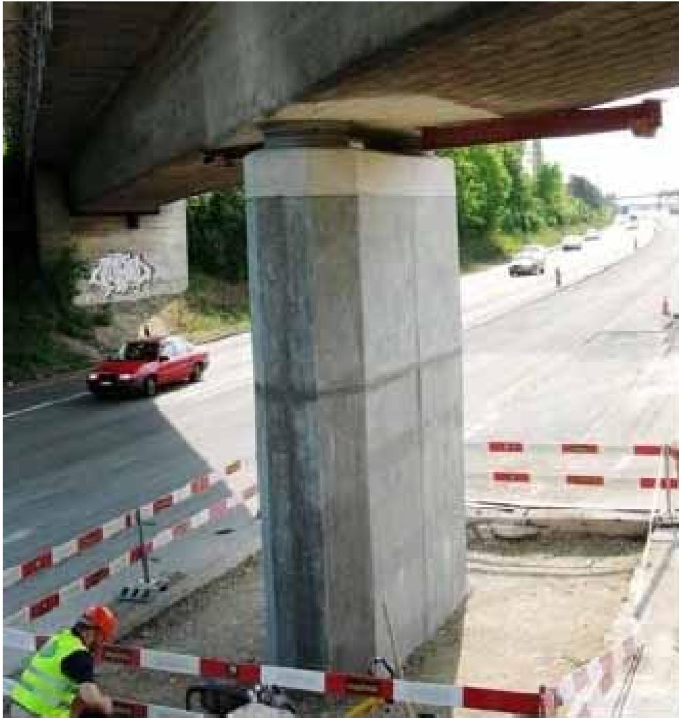
Bridge pier repair with UHPFRC at the A1, Killwangen (CH)
