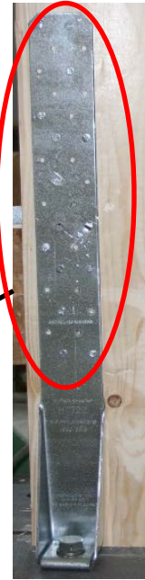
Hold-down with 12 \phi 4 \times 60 mm nails
