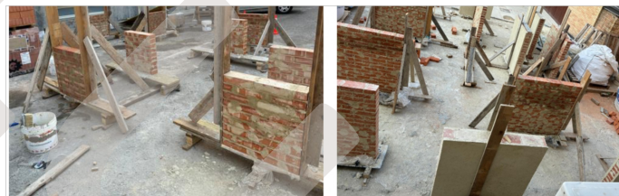
Masonry wall construction: (a) 0.60 m x 0.60 m, and (b) 1.2 m x 1.2 m.
