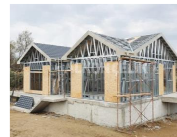
3. Shear walls with wood sheathing
