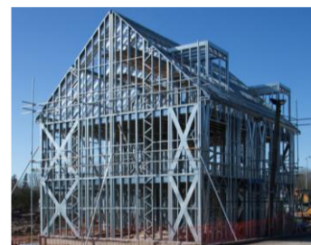
1. Strap-braced walls
