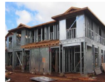
2. Shear walls with steel sheet sheathing
