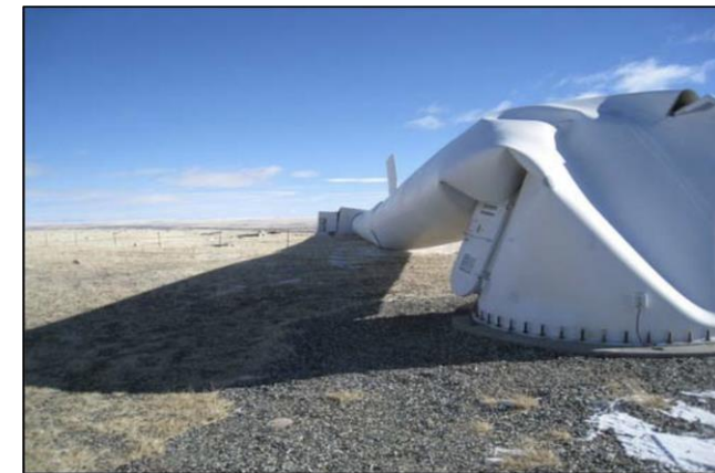
Section collapse at the base
